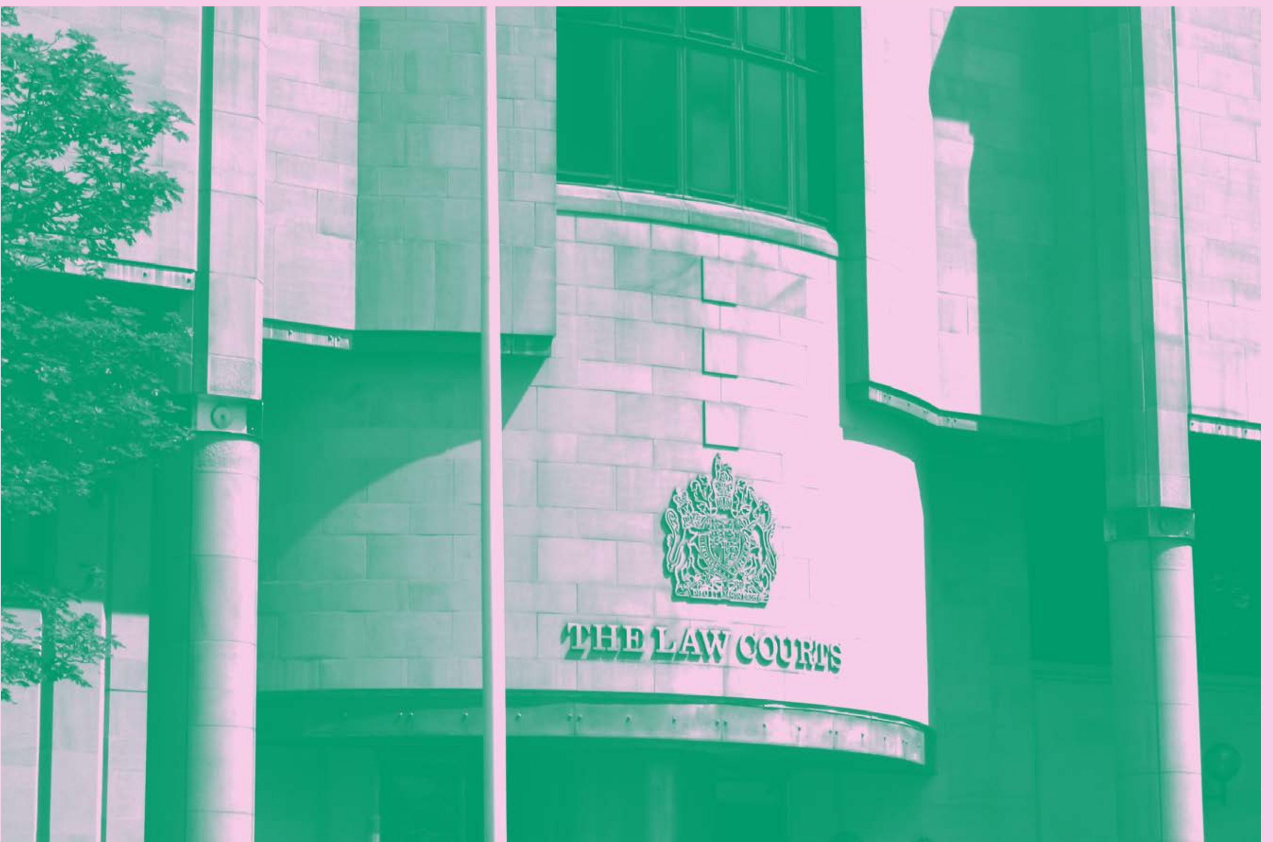
Crown Court Building
