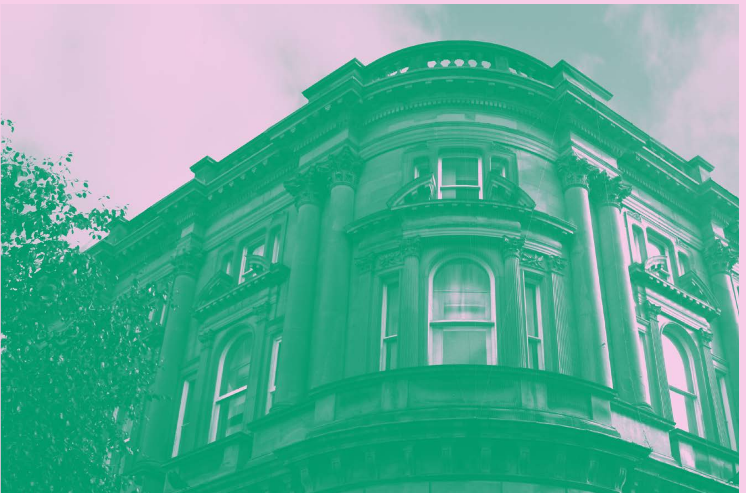
Bradford Banking Company building
